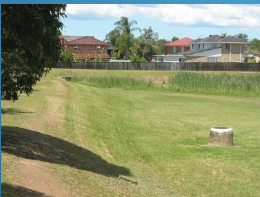
► Detention basin is an example of flood modification
