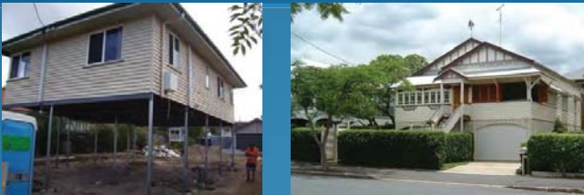
► House raising is an example of property modification
